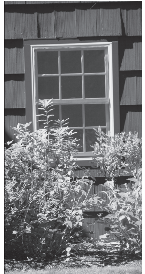
PLANTS AND gardens touching exterior walls of the home may provide the right environment for a termite colony.
